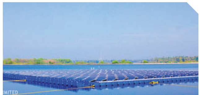
India's First Floating Solar Plant, Kerala - SPV Capacity: 100 kWp
