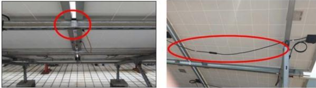
Figure 17: IMPROPER PV MODULES MOUNTING AND CONNECTION
